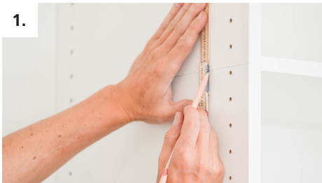
1. Mark the centre position of the shelf on the sides of the cabinet
