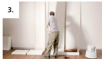
3. Place furniture side on base. The element is correctly positioned by the protruding screw
