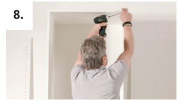
8. Join the furniture and subsequently fit the fixed intermediate shelves
