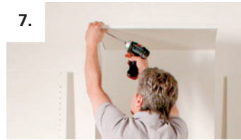
7. Screw front corner in place with a cordless screwdriver. This makes one-man assembly easy
